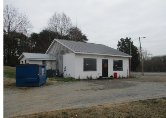
Picture 2: Existing building across from request location.
