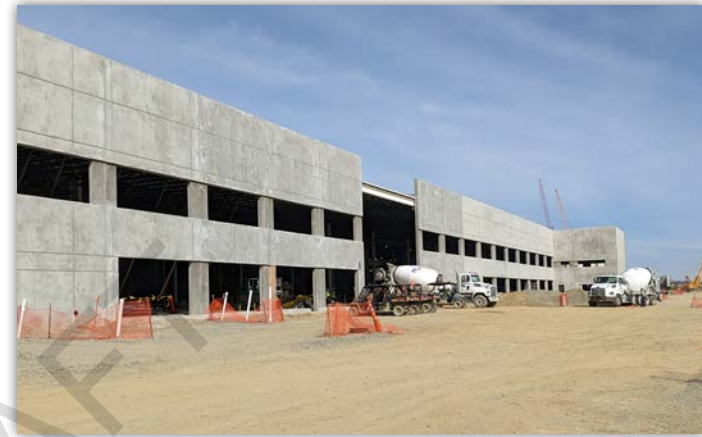
Image of Toyota Megasite under construction
