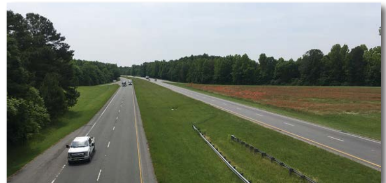
US Hwy 421 at Old Liberty Rd. Exit
