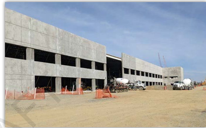
Image of Toyota Megasite under construction
