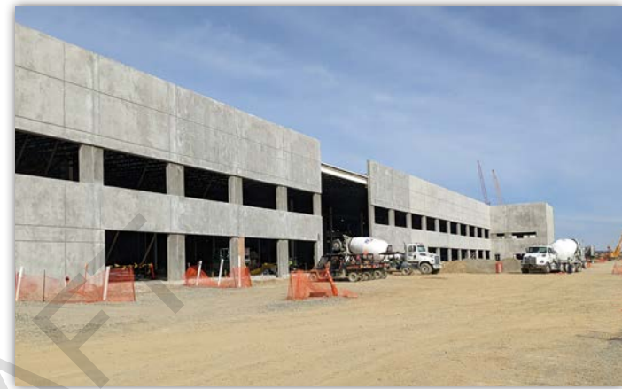
Image of Toyota Megasite under construction
