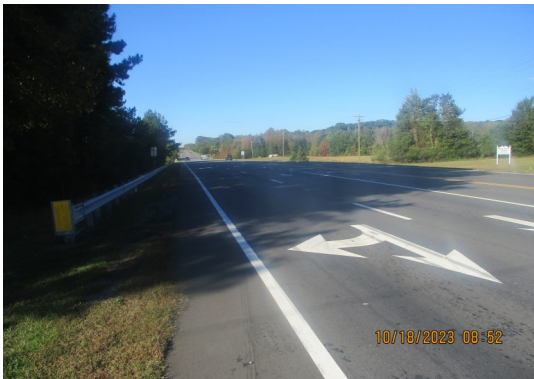
Picture 5: Request location on left as seen looking toward Crestwick Rd.
